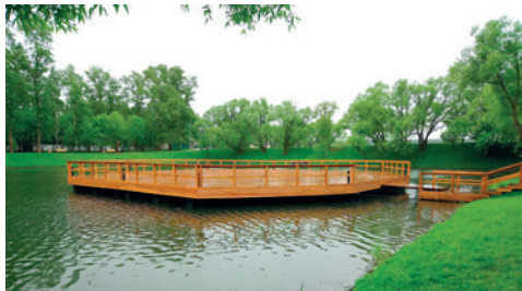
2018. Float modules of the B type were applied at the infrastructure development of the waterfront of the Meshcherskiy pond in Moscow.
