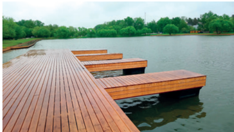
2018. Float modules of the B type were applied at the infrastructure development of the waterfront of the Meshcherskiy pond in Moscow.
